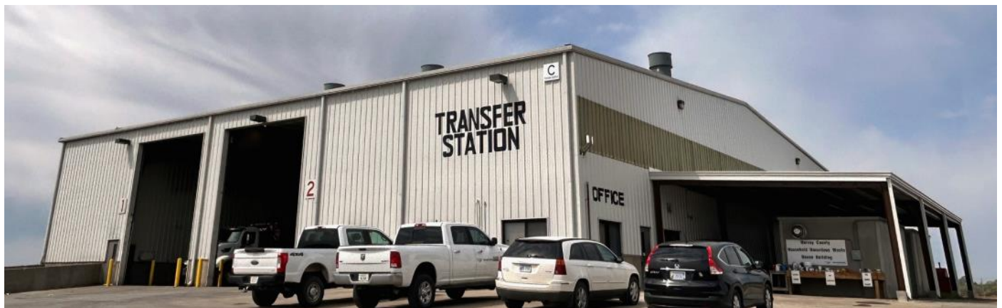
Harvey County Transfer Station Photo courtesy of Harvey County
