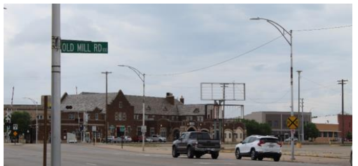
Old Atchison, Topeka, and Santa Fe Railroad Depot, now operated by BNSF
